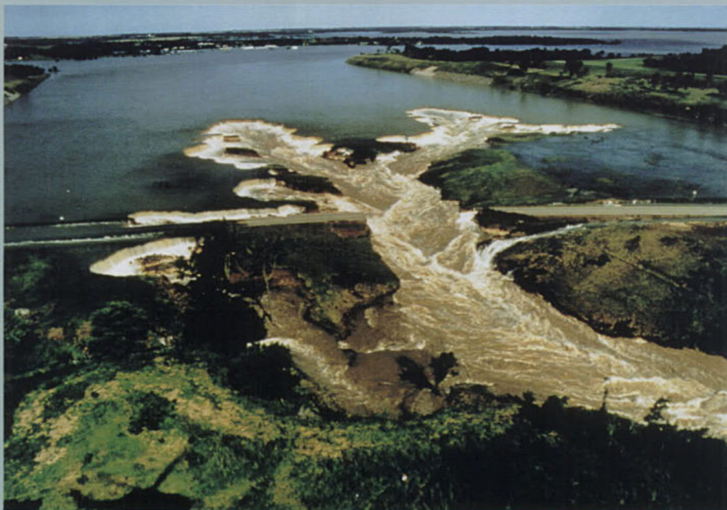
Milford Lake, KS Emergency Spill way Section 7/25/93
