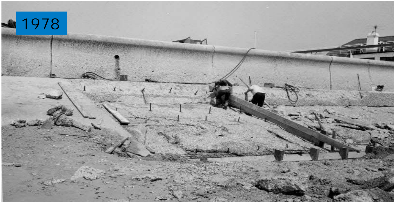
Major repairs required, as once again seawall is at risk of undermining.
