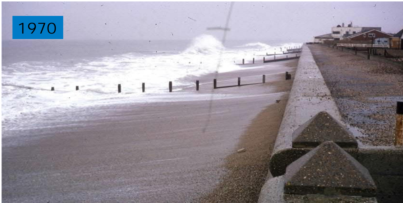
1970 Beach eroded. Early seawalls were undermined and replaced with bigger seawalls.
